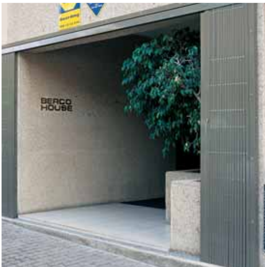
Trellidor Trojan retracts to allow entry
